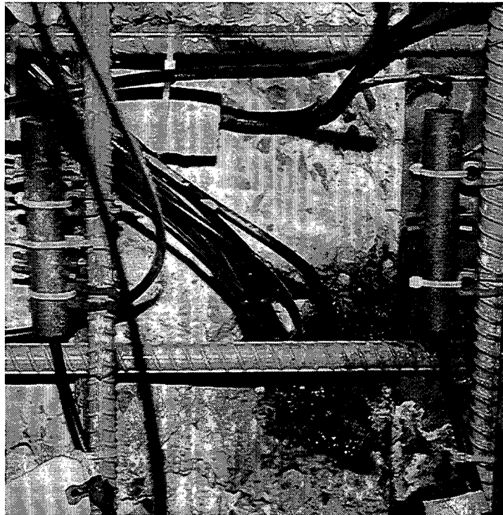
Graphite Half Cell and Rebar Probe in Place
