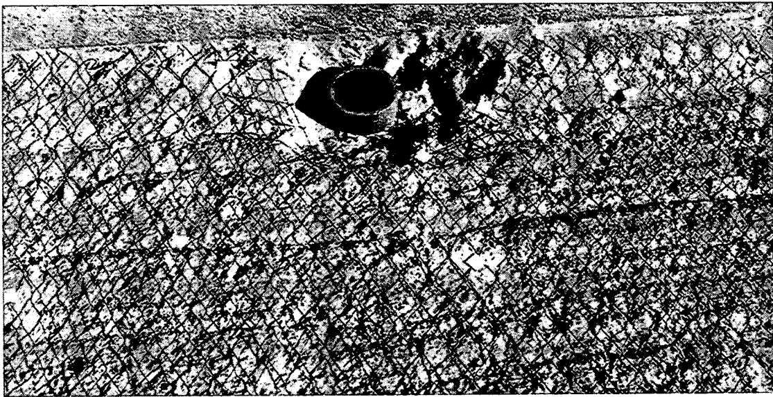
Anode Cut Around Drain Pipes to Ensure Electrical Isolation
