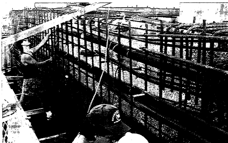
Post-tensioning Duct and New Steel in Place
