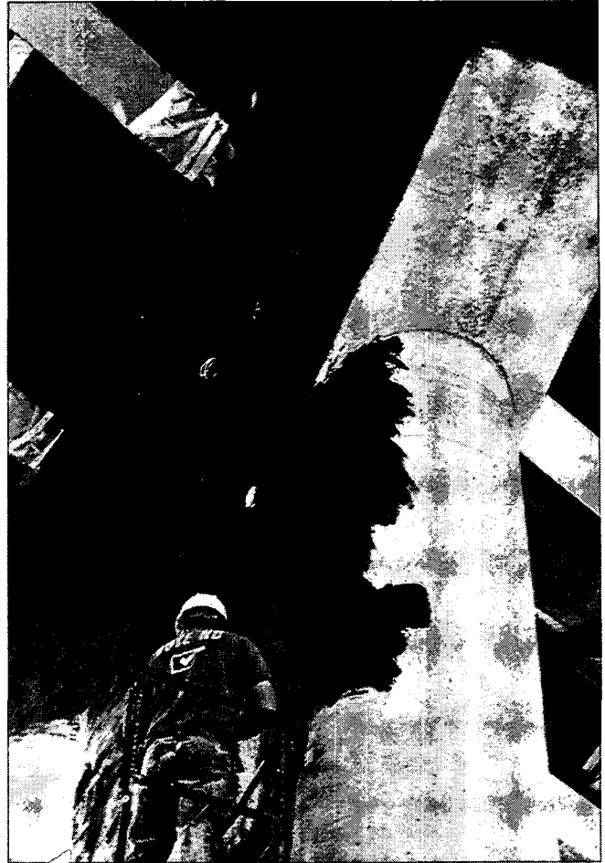
Application of Carbon Conductive Paint Anode
