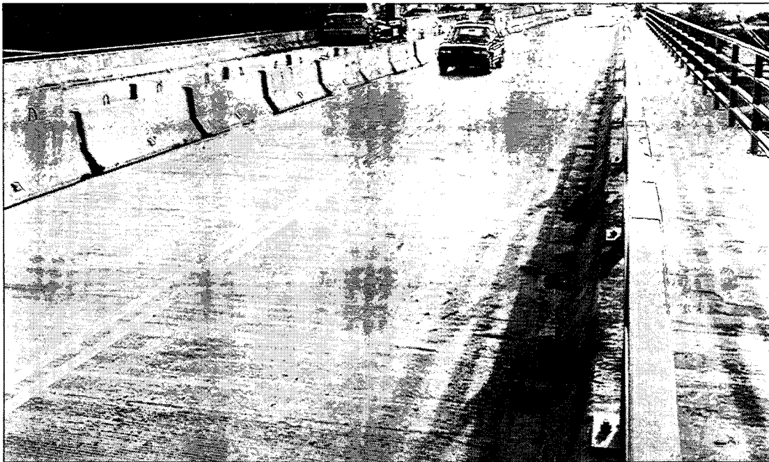
Structure Under Cathodic Protection in Use
