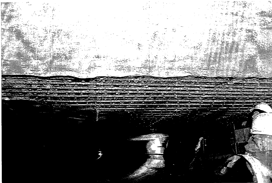
Mesh Ready for Shotcreting (Finished shotcreted surface in the Foreground)
