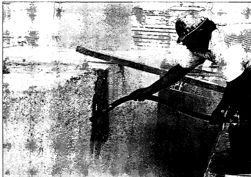
Sandblasting in Progress
